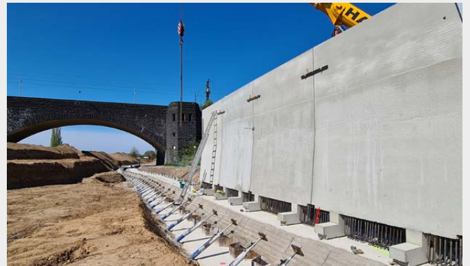
The retaining wall is made up of precast concrete elements
